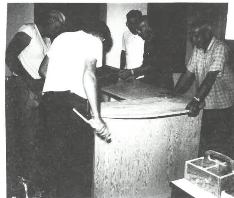
BUILDING KITCHEN CABINETS
